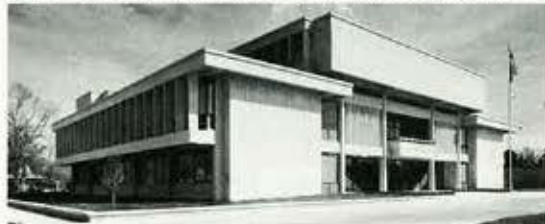
Tangipahoa Parish Courthouse, Amite, La.
